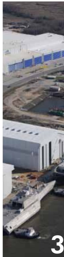
3 MMF UPGRADE COMPLETE
